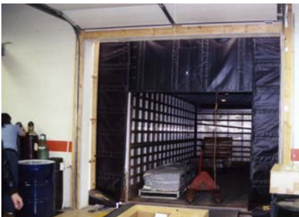
RIGID FRAME INSIDE LOOKING OUT
