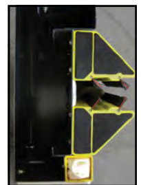
Thermal breaks in side column along with quad seals (red highlights)
